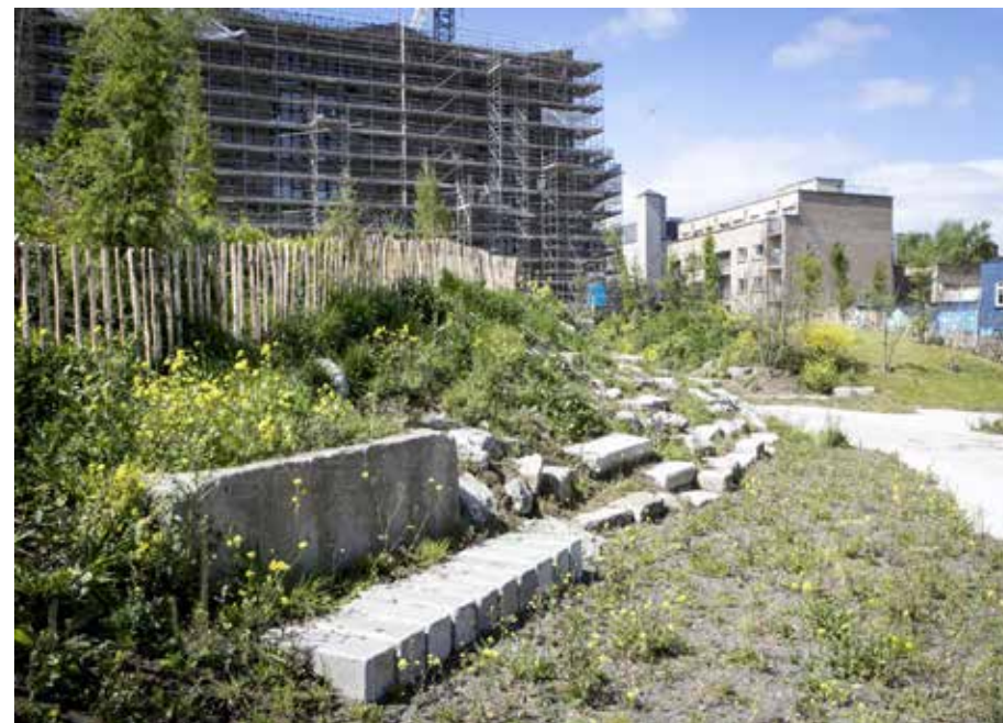
Reuse of crushed concrete as growing medium and playfu elements. Bridgefoot Street park Dublin
