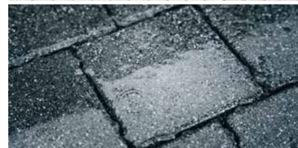
Permeable paving for car and cycle parking
