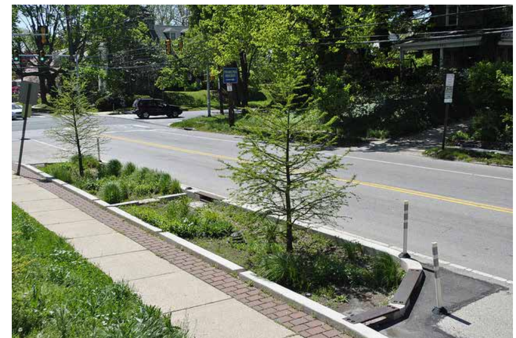
Bioretention tree pits
